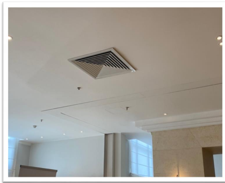
Figure 1: A picture containing 4 systems which are in Place at one of the Five-Star Hotel; Fire Curtain which is hidden in the ceiling and upon activation protects the staircase, Sprinklers protecting the fire curtain, HVAC system outlet and a smoke detector.
