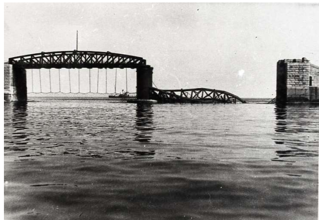
Fig. 1.1 The breakwater viaduct before the attack (left), with one span, collapsed immediately after the attack (right). Note the fallen girders of the outer span creating a further obstruction to the passage. The
