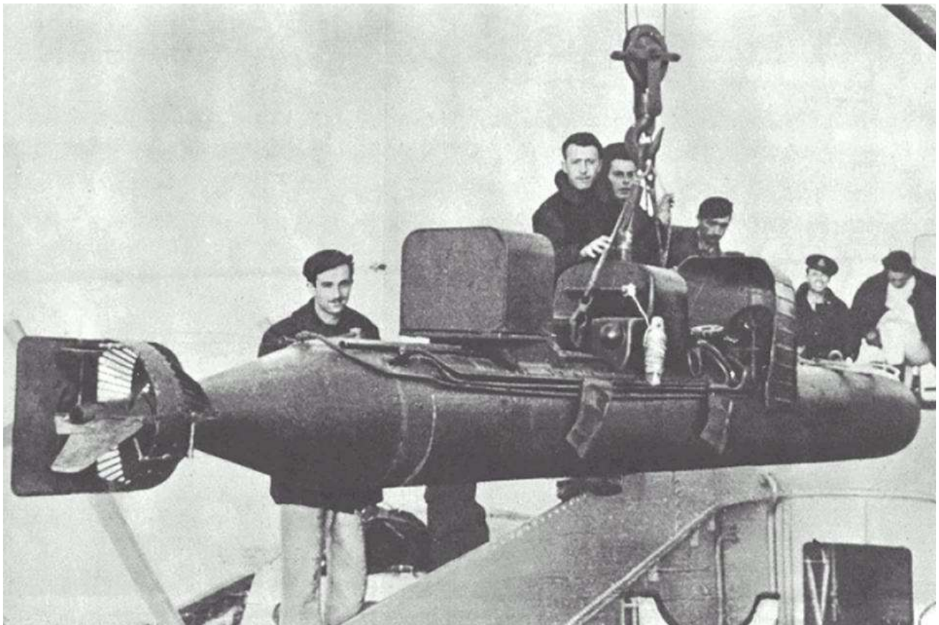
Fig. 2.5. A midsize submarine of the type developed by Teseo Tesei which was used in the attack on Grand Harbour. These were slow-running manned torpedoes called SLC nicknamed Il Miale by the Italians. (Maj Tony Abela, The Times of Malta , 23rd July 2016, Photo: Vincent P. O'Hara, Enrico Cernusch)
