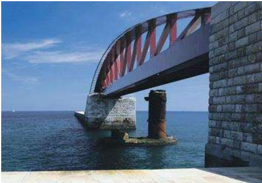
Fig 1.2 a & b. The remains of the central legs that used to support the viaduct linking St Elmo Point to the breakwater. In 2012 a new bridge was built linking the span. (Maj Tony Abela in The Times of Malta 24 th July 2016).
