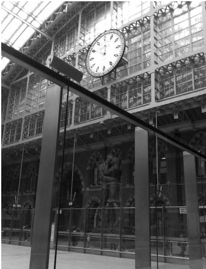
Fig. 10.5. St Pancras Station platform. (Pictures © Peter Robinson.)
